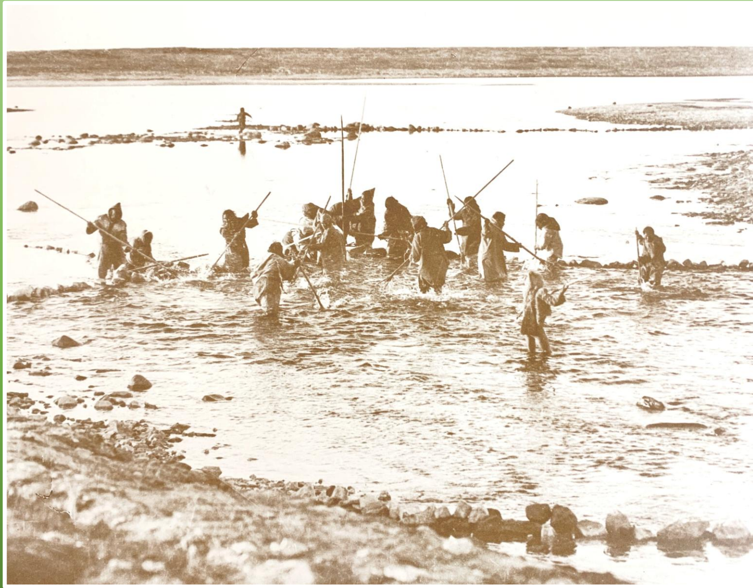
Fishing at a stone weir in river. Stone gates are opened to allow fish to enter, then closed, and people spear them with long fish spear (Inuktitut: kakivak). Archival photo from the central Arctic coast.
